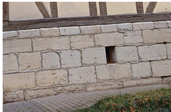
Natursteinsockel in Windeberg
